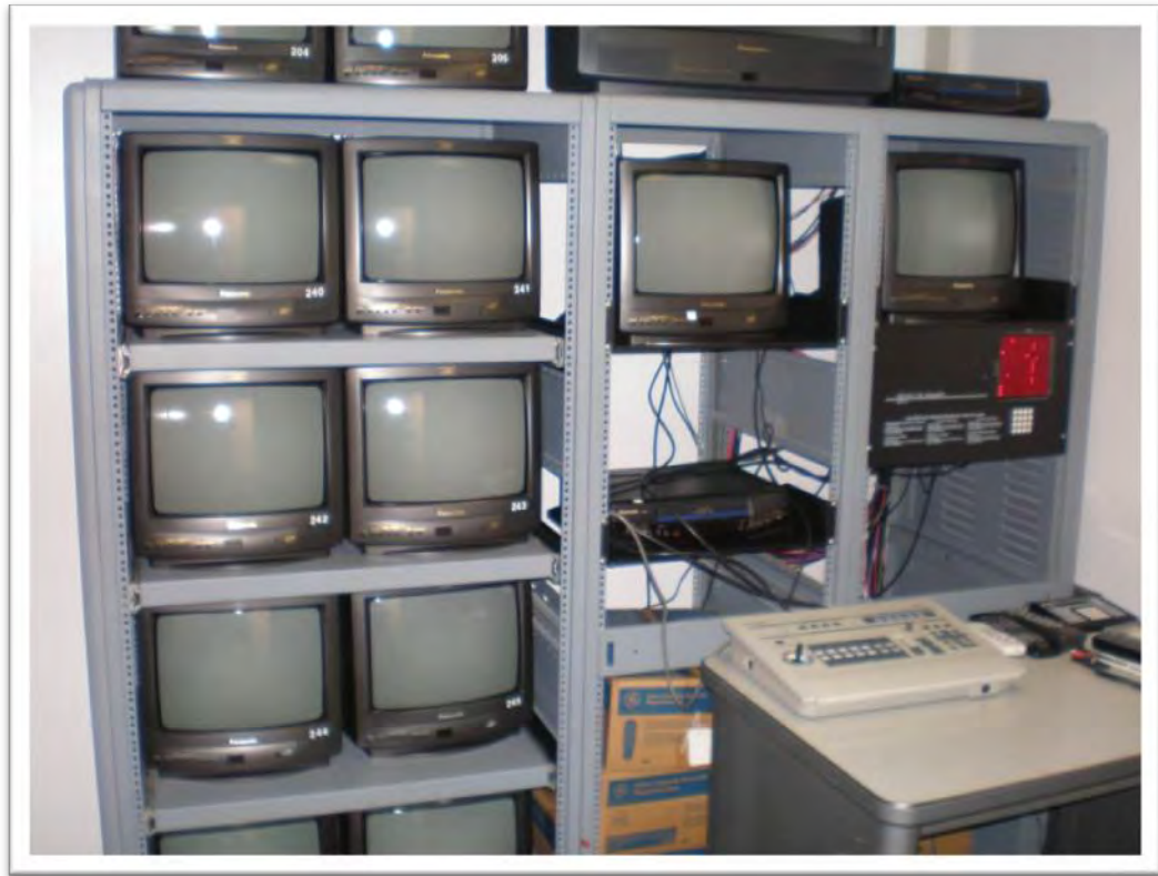
Figure 1: Original VHS Closed-Circuit Control Room.
